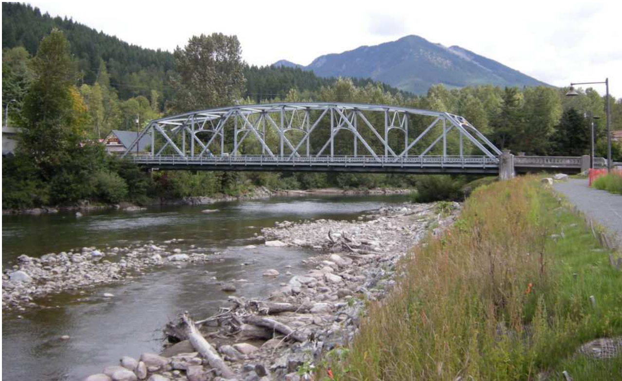
The Bridge to the Town of Skykomish from Highway 2 is one of the most notable features in this town.
